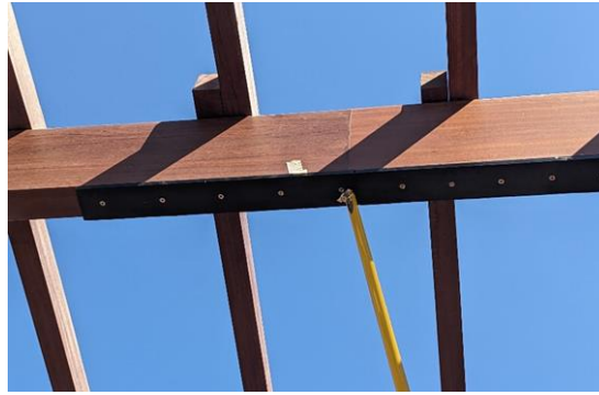
Figure 1 Application of glued-in rod joint system in long-span timber beams.
